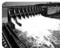
A dam used to generate electricity
