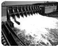
A dam used to generate electricity
